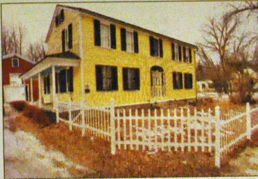
This Federal-style home, built in Bridgton in 1828 and once called Far Hills for its view of the Oxford Hills, is on the National Register of Historic Places.
